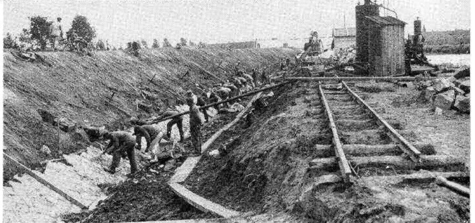
Curange-Beringen Section. Rubble work after lowering the water strata.
